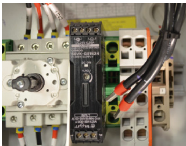
Figure 10 Wiring box for PVI-3.0/3.6/3.8/4.2 and PVI-5000/6000
